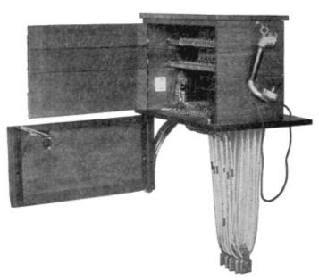
Fig. 304. Sectional Switchboard—Wall Type View full size illustration.
