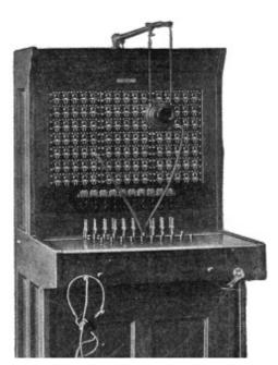
Fig. 299. Magneto Switchboard, Target Signals (partial) View full size illustration.
