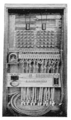
Fig. 295. Upright Magneto Switchboard—Rear View View full size illustration.
