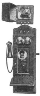
Fig. 191. K.B. Lock-Out Station View full size illustration.
