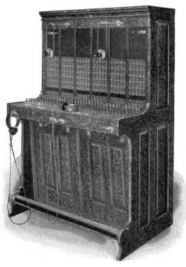
Fig. 301. Dean Two-Position Switchboard View full size illustration.
