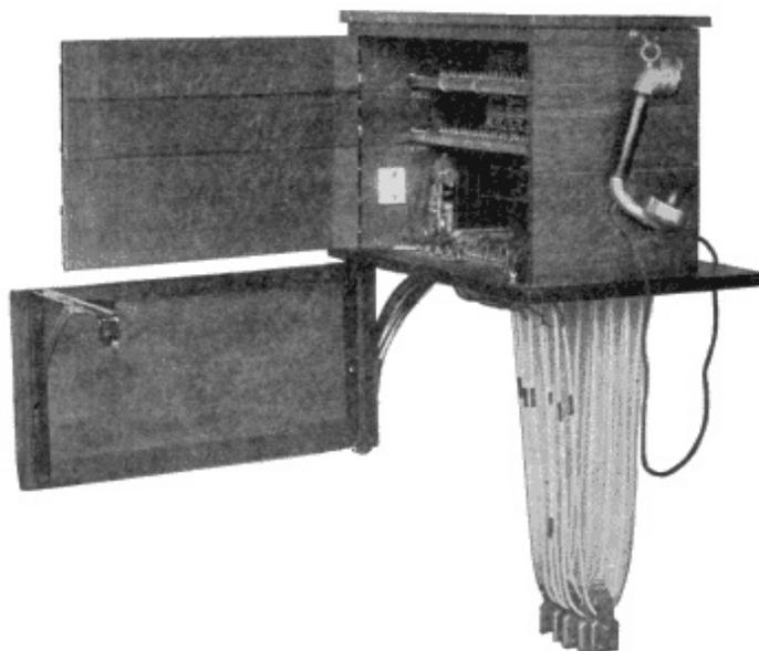
**Fig. 304. Sectional Switchboard—Wall Type**
