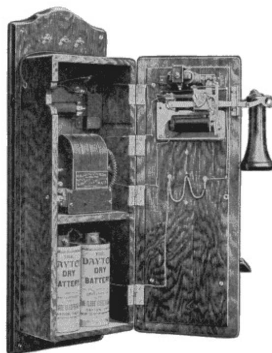
**Fig. 190. K.B. Lock-Out Station**
