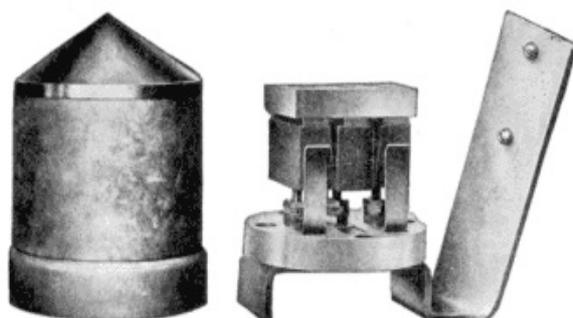
**Fig. 210. Western Electric Air-Gap Arrester**
