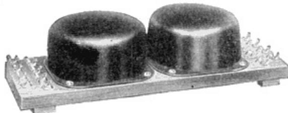
**Fig. 113. Toroidal Repeating Coil**
